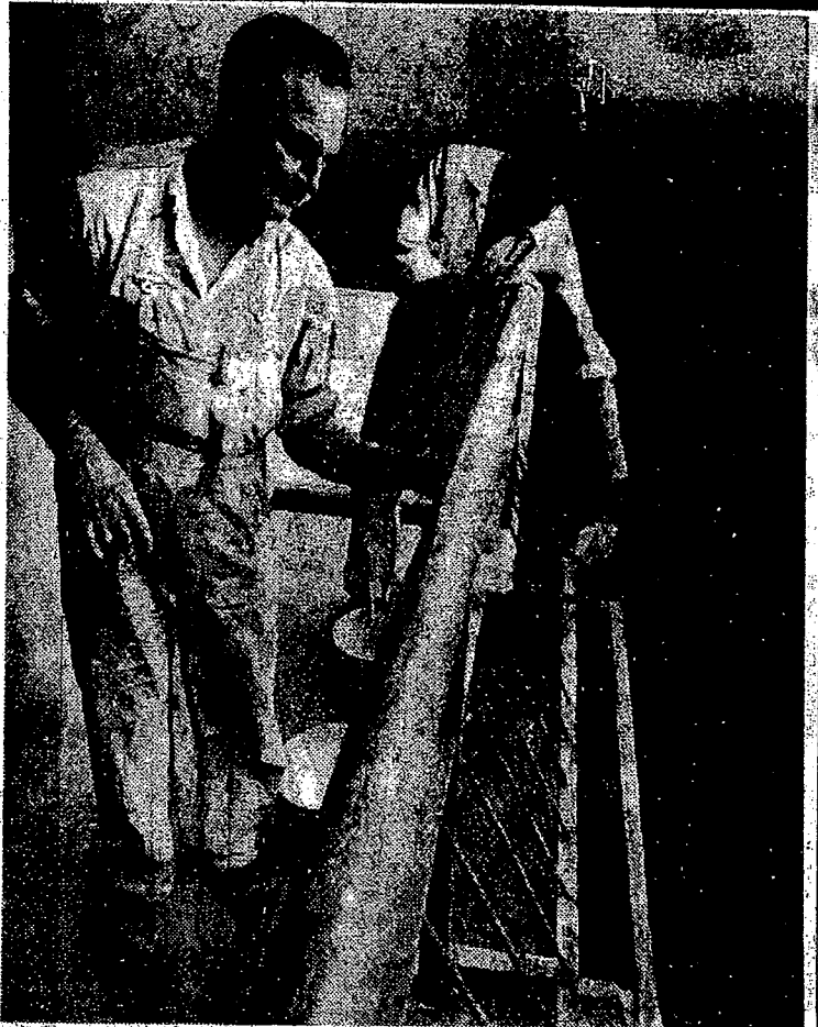
TWELVE FLOORS up, painters Arthur Scheller (left) and George Mussen put finishing touches to a balcony on Torbreck apartment block.
